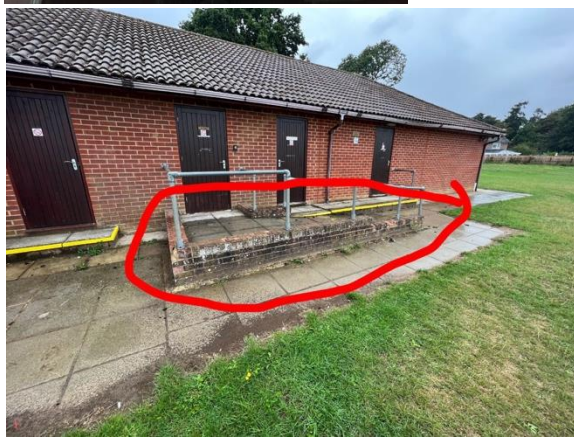
Picture 3 – Replace missing bricks, remove broken bricks and re cement.
