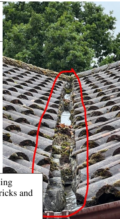
Picture 1 & 2 – Rake both valleys of old cement and re cement valleys both sides.
