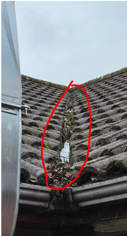
Picture 1 & 2 – Rake both valleys of old cement and re cement valleys both sides.
